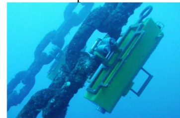
FIGURE 2: INCLINOMETERS INSTALLED ON TOP CHAIN. COURTESY: PULSE [5]
